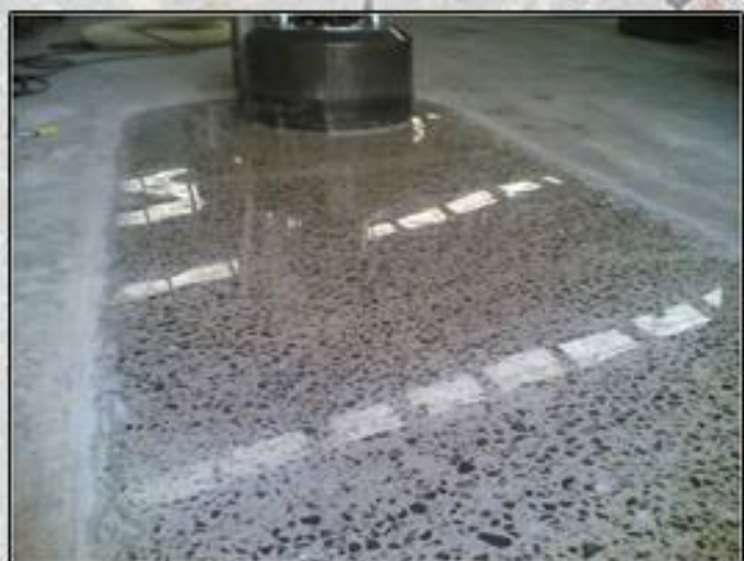
(Concrete Polishing)
